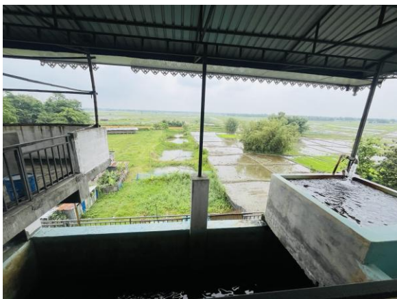
Photo 22: Observation of hatchery infrastructure and water supply system during the consultant visit.
